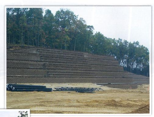
Public safety was a big concern. Walltek designed and engineered the wall to exceed specifications under this stress. Each tier measures 7-feet in height and each is spaced 5-feet apart—as independent walls. At the highest point, the wall's height is an imposing 42 feet. Much lower sections of the wall run the perimeter of the school grounds.
